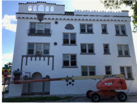
NEW ROOF COMPLETED!
